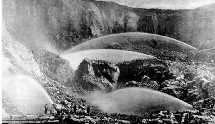
Figure 8. Hydraulic mining in the Sierra Foothills.
